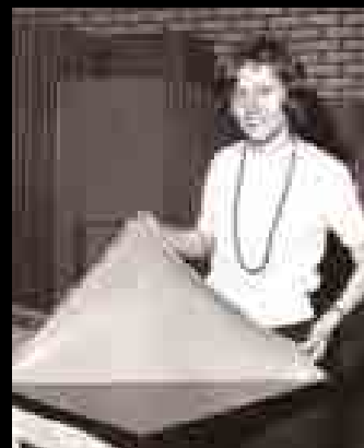
Gulvie Tye unmarks some early stainless steel sinktops destined for the Barbican Estate in London. Architects, Chamberlin Powell & Bon were seeking ultimate efficiency and space-saving. A place where space for a kitchen was most at a premium was on board a boat, so yacht designers, Brooke Marine, were brought in and GEC Anderson were able to meet their specification precisely.
