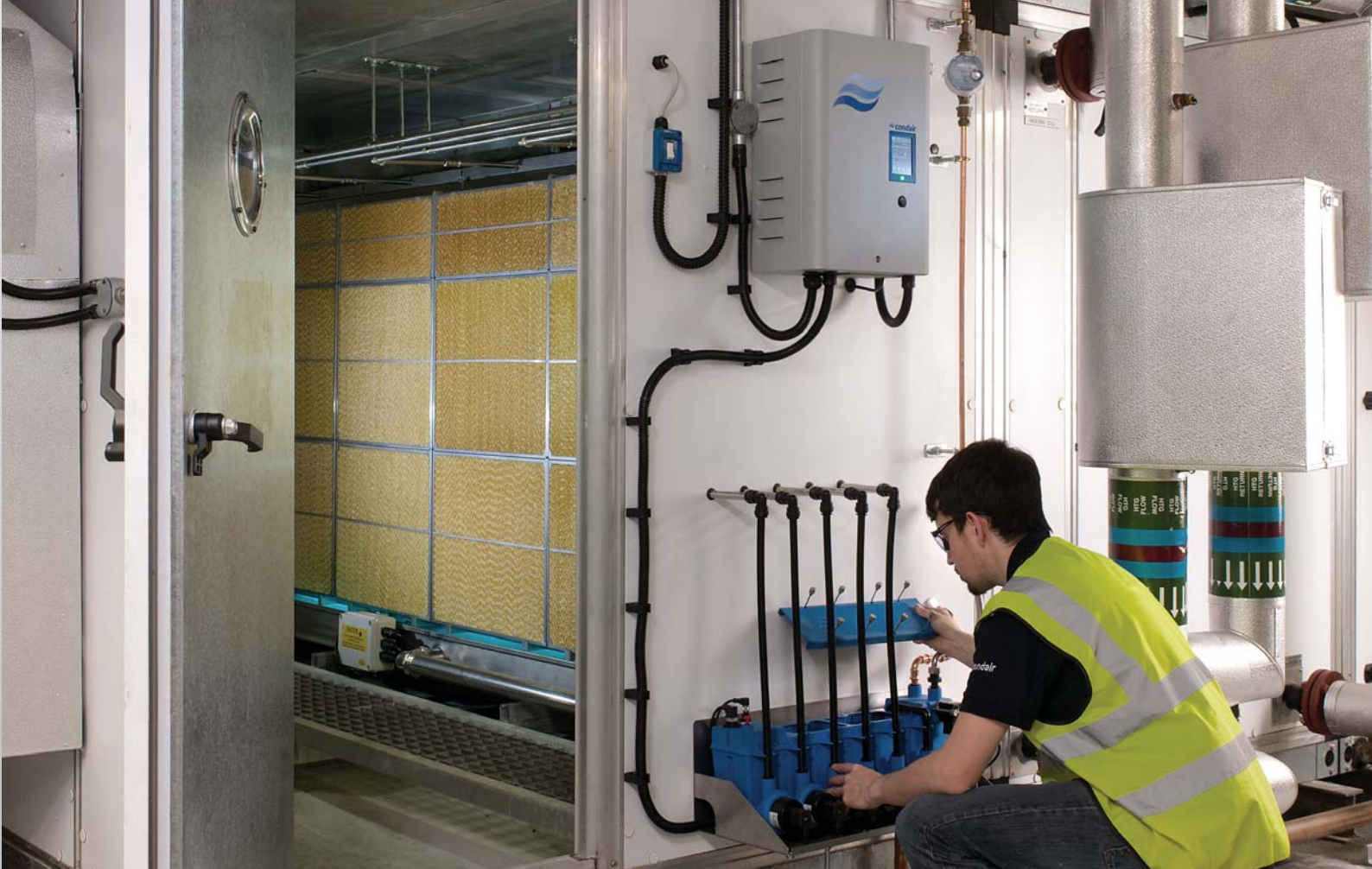
Condair ME with externally mounted hydraulic unit
