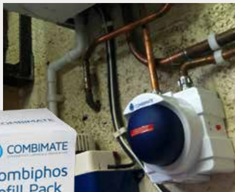
A protective outer cover is fitted to complete Combimate installation.
