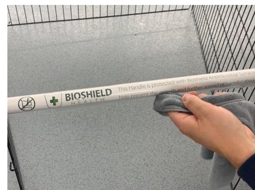
Step 6 – Work your way around the bottom of the handle, firmly pushing the kit down to push out any air.
