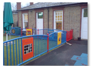
These railings are manufactured from 50mm round steel tubing with 25mm tubular vertical bars, they have coloured polyethylene infill panels. Available with a range of graphics and activities engraved on one side.
