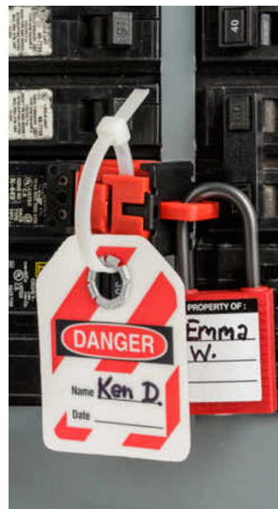
Can be secured with cable ties and/or a safety lock
