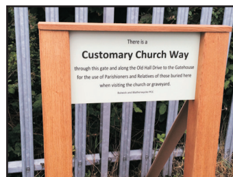
F10. Side mounted posts and weather board.
