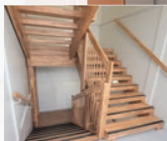
Internal staircase with landing platform
