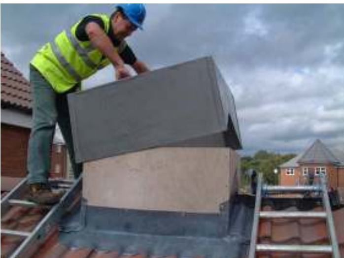
Lead effect GRP skirt being put into place over ridge box.
