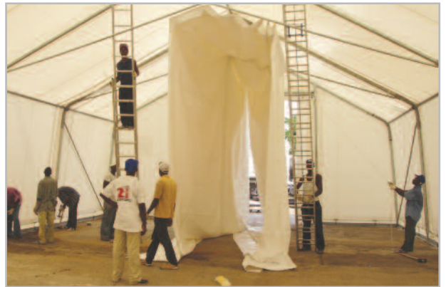
Inner skin being installed in a 10m(32.8') span THAB delivered to the UN in Sudan
