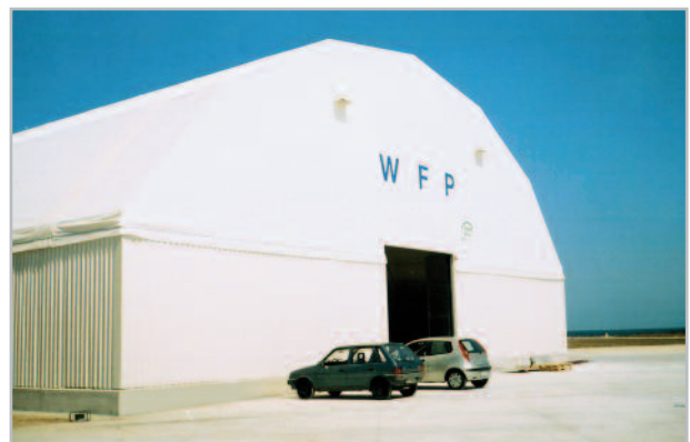
20m(65.6') span NV type building and 10m(32.8') span THAB type shelter supplied to UN in Congo
