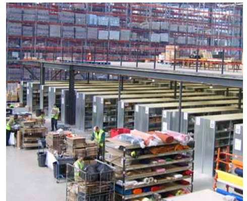
Mezzanine beams, stairways and handrails are designed to conform to the requirements of the latest regulations.
