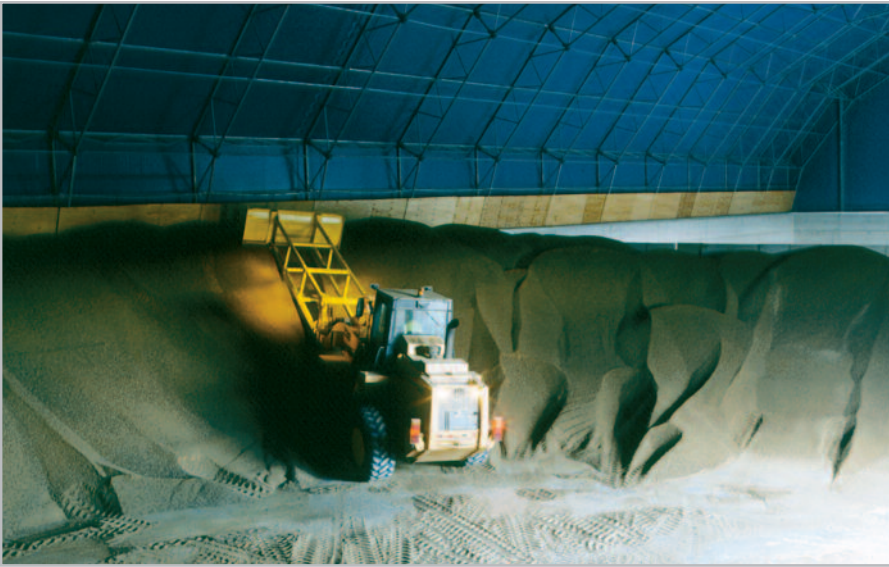
Left: Bulk Storage, Workington, UK. 82' (25m) span NV (Norway Vertical) type structure with intergrated concrete retaining walls to hold bulk material.
