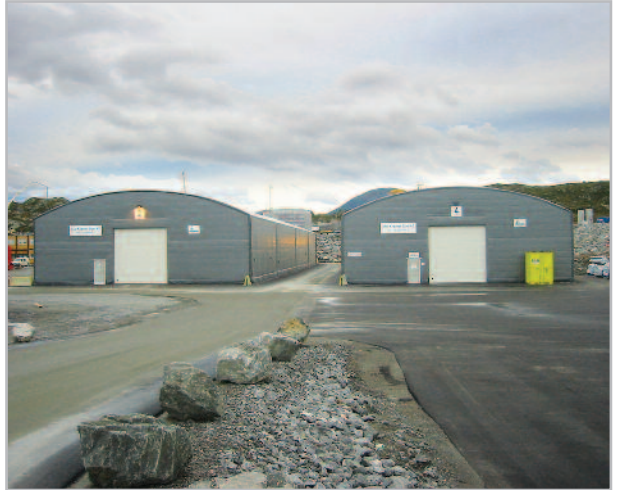
Right: Aker Solutions, Stord, Norway Aker Solutions land-based insulated Thermohall workshops near Bergen, Norway. The Thermohalls provide fully functional, forward-based maintenance facilities for Aker's North Sea Oil and Gas extraction activities.
