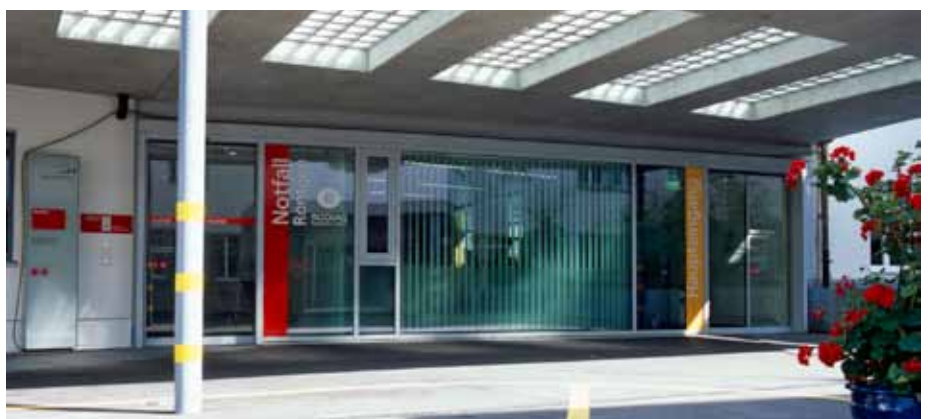
Main and emergency entrance of Zimmerberg hospital, Switzerland, single-sided telescopic sliding doors
