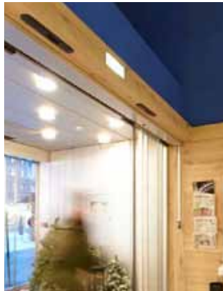
Fire proof sliding door (EI30) towards the corridor, Vienna, Austria
