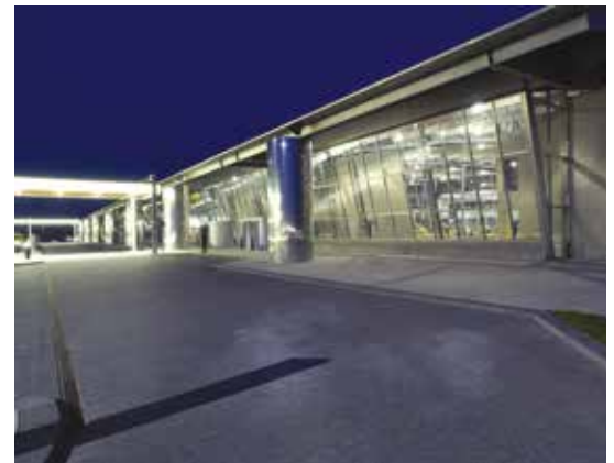
Automatic doors, facade, BLL
