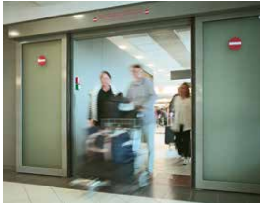
Automatic fire protection door, baggage claim, LYS
