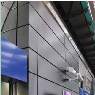
interior wall linings 4-5
