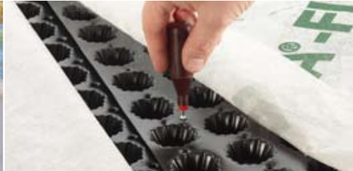
Joining sheets with DELTA®-FLORAXX connecting elements.
