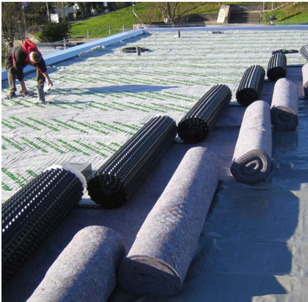
Fast, cost-efficient laying thanks to the integrated geotextile.
