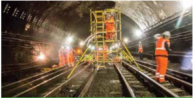
RESIN INJECTION - LONDON UNDERGROUND
