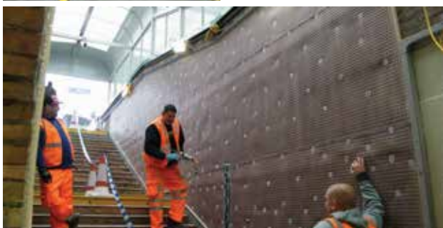
DAMP PROOFING - LONDON UNDERGROUND STATION
