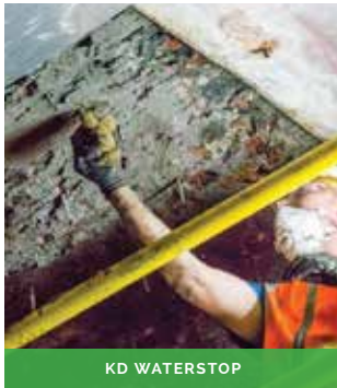
RESIN INJECTION - LONDON UNDERGROUND
