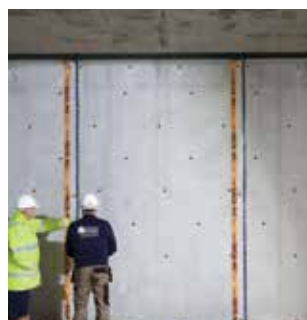
ON SITE SUPPORT
