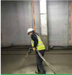
NB1 SPRAY APPLICATION
