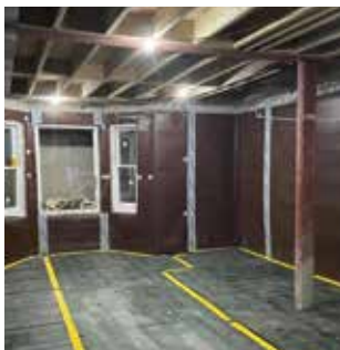
TYPE C WATERPROOFING & GROUND GAS PROTECTION
