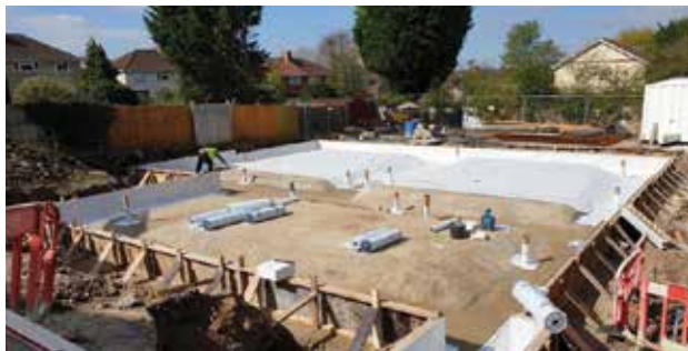
DELTA DUALPROOF INSTALLATION
