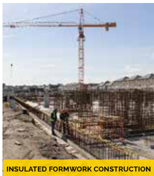
INSULATED FORMWORK CONSTRUCTION
