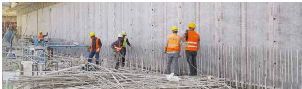
APPLICATION OF DELTA AMPHIBIA SYSTEM ON REGULARIZED DIAPHRAGM WALLS
