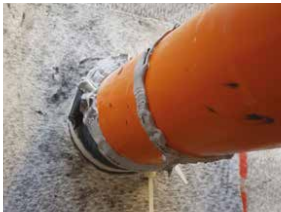
SEALING PENETRATION WITH HYDRO-EXPANDING MASTIC AND DELTA AMPHIBIA SYSTEM
