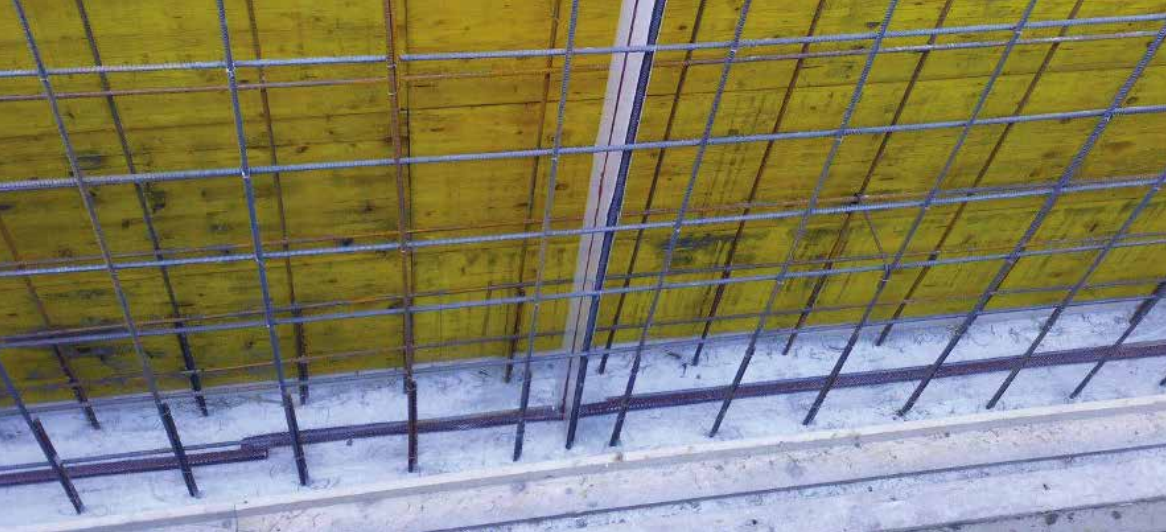
APPLICATION OF SELF-SEALING STRUCTURAL CRACK INDUCER BREAK
