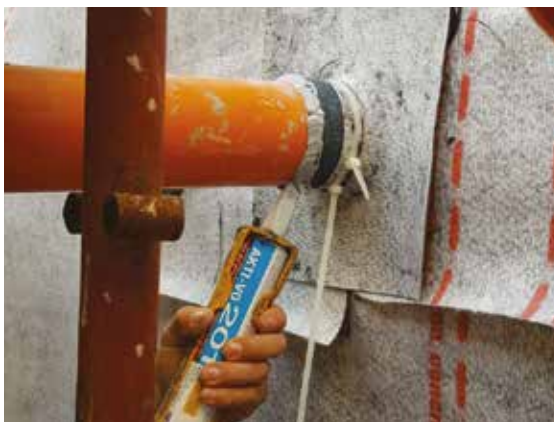
02.1/02.2 | DELTA AMPHIBIA INSTALLED ON SLURRY WALLS/EXISTING STRUCTURES- SEALING OF PENETRATIONS
