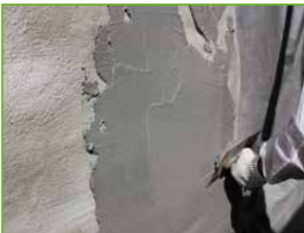
4. Apply the first coat by flat trowel, tooth trowel, or appropriate spray equipment.
