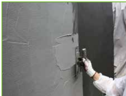
5. The application of the second coat is already possible after approx. 3-4 hours.
