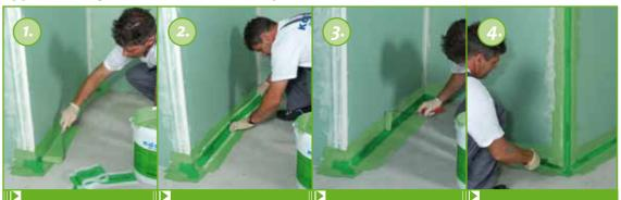
Apply a covering coat of KÖSTER BD 50 to the area where the KÖSTER BD Flex Tape K 120 is going to be installed.
