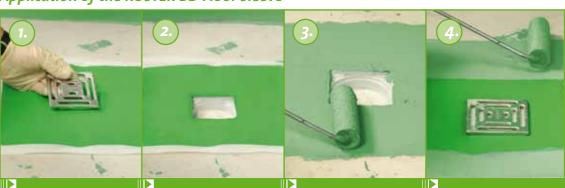
Position the KÖSTER Floor Sleeve over the floor drain on which it is applied.
