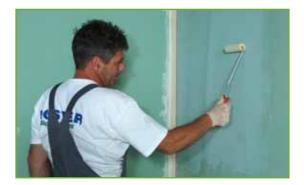
KÖSTER BD 50 Primer is applied to the substrate by roller or brush. Different substrates require different consumptions of the KÖSTER BD Primer. For priming gypsum board, dilute KÖSTER BD 50 Primer with water in a ratio of 1:3. Consumption of that mixture is approx. 240 g / m². For details on other substrates, refer to the technical data sheet of KÖSTER BD 50 Primer.
