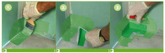
Apply a covering coat of KÖSTER BD 50 Embed the KÖSTER BD Inside Corner to the area in the inside corner where the KÖSTER BD Inside corner is going to be installed approx 10 cm up onto the wall and 10 cm onto the floor.
