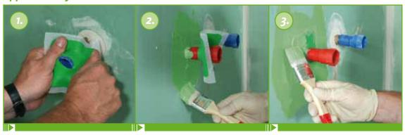
Slide the KÖSTER Wall Sleeve over the pipe penetration.
