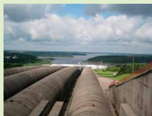
Water power plant, Lithuania
