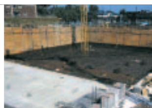
DELTA®-GEO-DRAIN Quattro protects compression-sensitive waterproofing.
