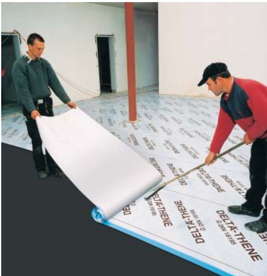
Large surfaces can be sealed easily and quickly with DELTA®-THENE.
