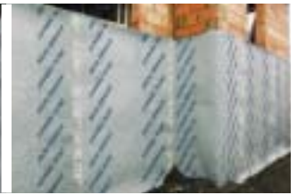
Permanent filtration and drainage.
