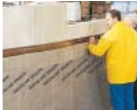
DELTA®-NP DRAIN ensures reliable drainage.
