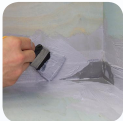
3. Apply Pre-formed Corners (internal or external)
