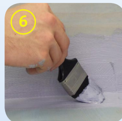
6. Finish by applying 2-3 coats of Compound over the entire area
