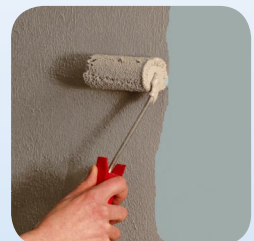
6. Finish by applying 2-3 coats of Compound over the entire area
