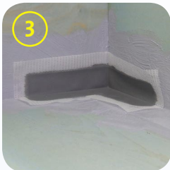
3. Apply Pre-formed Corners (internal or external)
