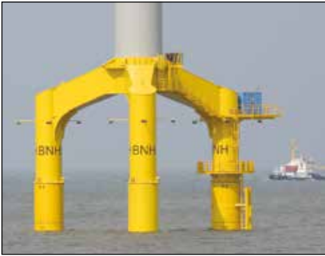
▲ Offshore wind turbines levelling: Enerpac's synchronous lifting system provided the solution for levelling the supporting cross pieces for 80 wind turbines.
