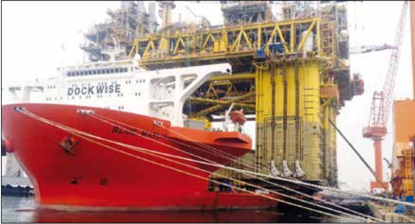
▲ The superlifting and launch of a 43.000-ton floating oil production system in Malaysia for the Gumusut-Kakap offshore field has set high benchmarks for safety through its use of sophisticated EVO-Series synchronous hydraulics to lift, balance, weigh and smoothly launch massive resources structures.
