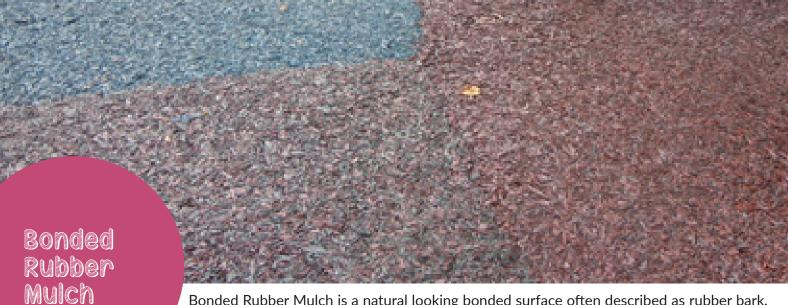
Bonded Rubber Mulch is a natural looking bonded surface often described as rubber bark. Laid in-situ, it is a durable and environmentally friendly safety surface containing 100% recycled rubber.
