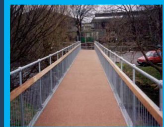
Fig 18: HFS - Metal Deck Bridge
