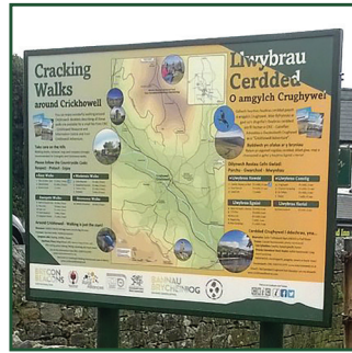
VI. GRP sign with vertical aluminium posts & frame
