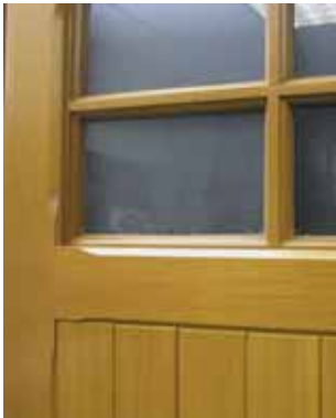
Glazing details of a Sherwood Southwell showing glazing bar details, the windows in this door are a solid window sash inserted into the door panel as shown
