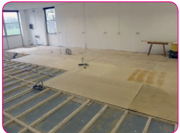
new floor which had to be installed
