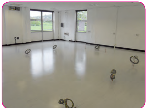
the new floor with all services ready for furniture and benching
