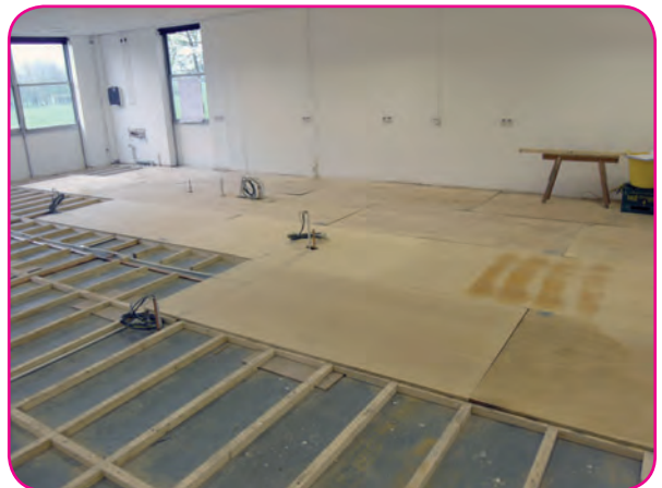
new floor which had to be installed
