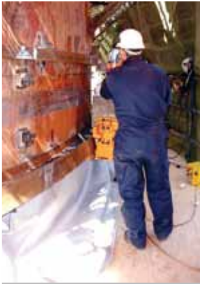
7. 'C' plate brackets fully welded and setting machine on the rail
