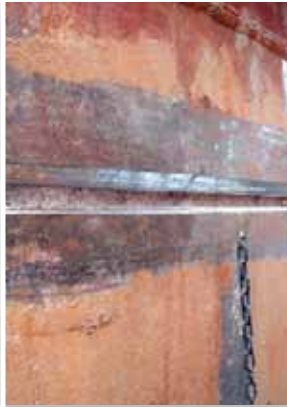
9. Finished prep showing refractory wall
