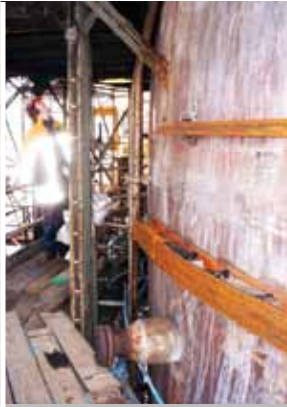
4. Rail positions showing non-removable obstructions
