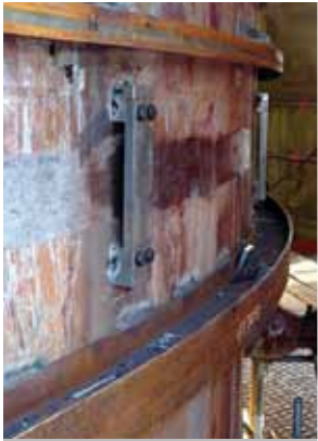
6. 'C' plate brackets tacked over cut line area
