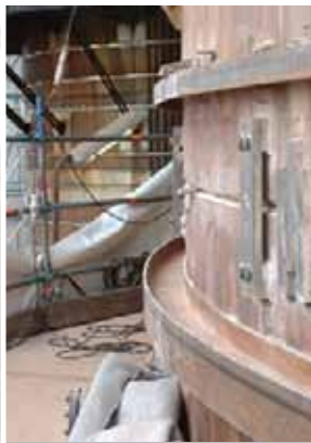
14. Prep completed. 'C' plates and alignment plates fitted
