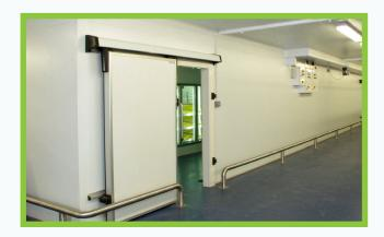
Volt free contacts from a refrigerant leak detector and/or a personnel entrapment alarm can be wired directly to the door alarm to activate these features.
