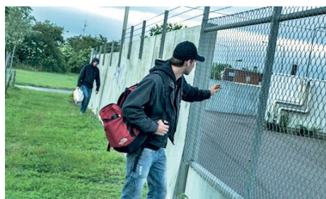
PERIMETER INTRUDER DETECTION
