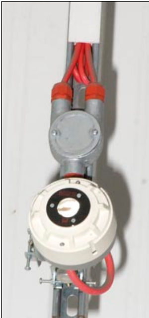
Figure 37 Smoke detector
