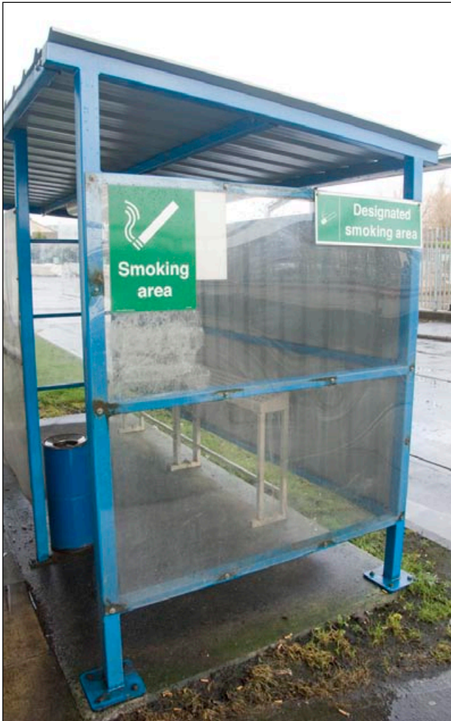
Figure 21 Designated smoking area away from the chemical store
