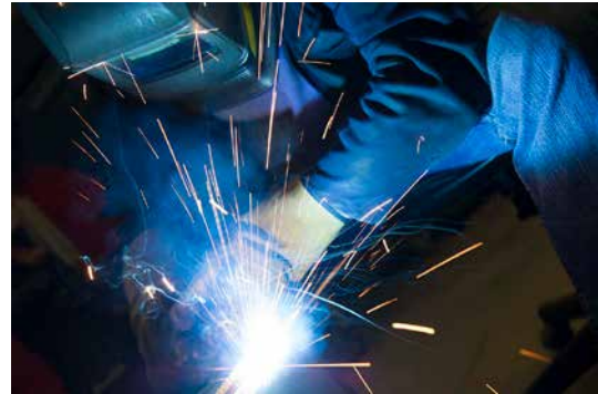
On-Site coded welders
