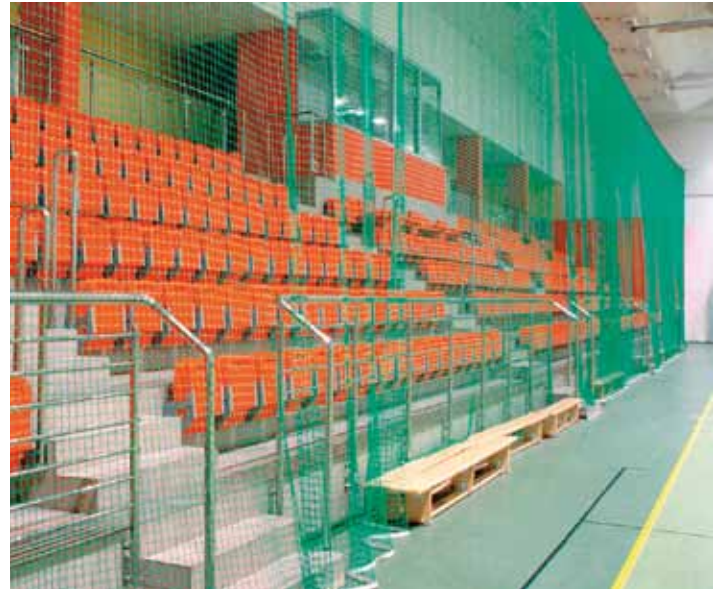
Spectator Area Protection Netting
