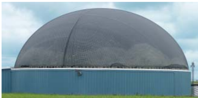
Outer net of a biogas installation in the USA with safety net made from high-strength polypropylene, approx. 5 mm dia., mesh size approx. 45 mm
