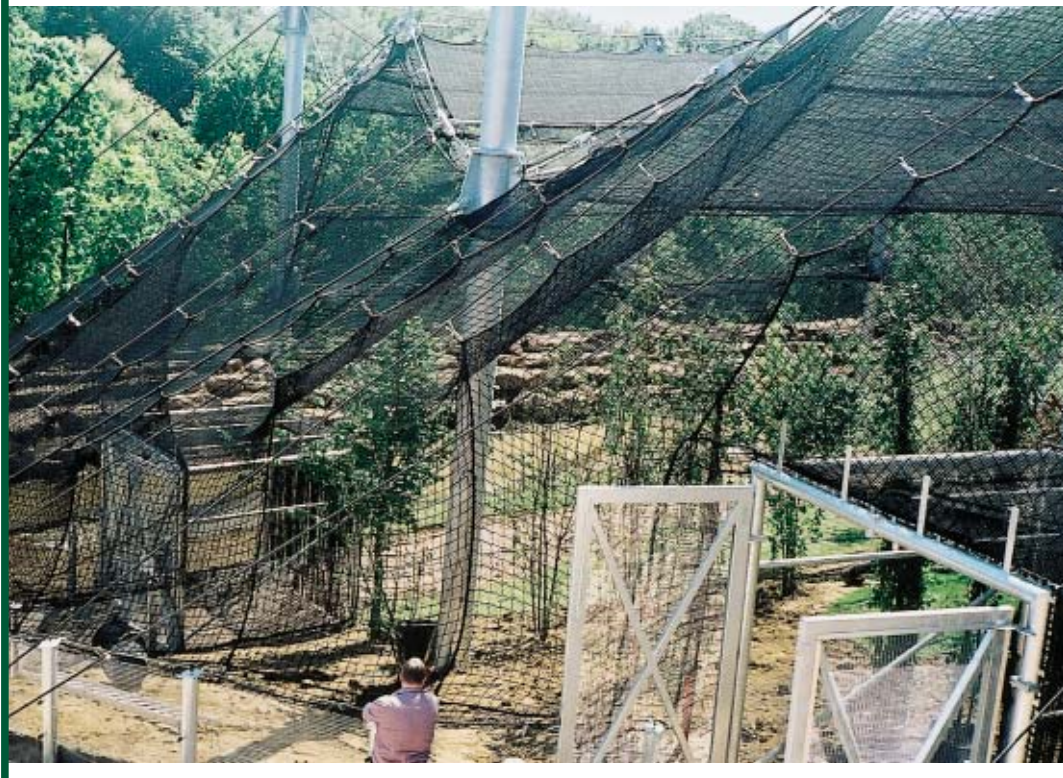
Installation by Huck-Torimex, Mondo Verde bird park in Landgraaf, the Netherlands.
