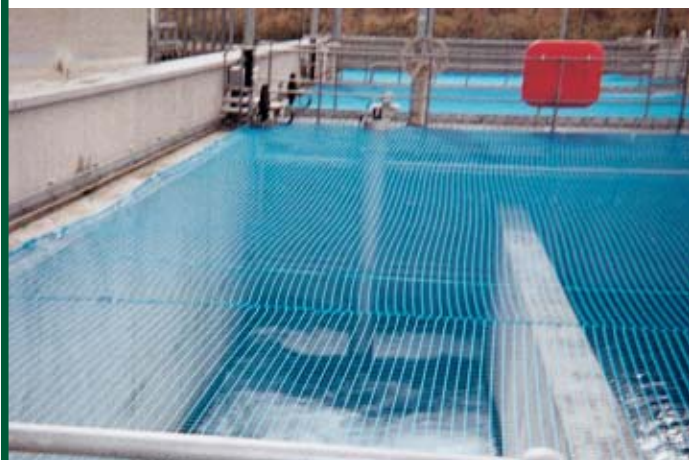
Sewage treatment safety nets
