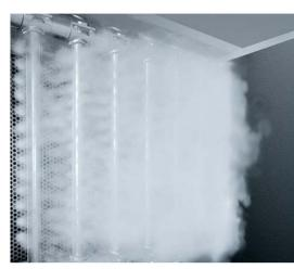
The hot dry steam is absorbed quickly and uniformly by the air stream.
