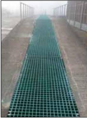
50mm thick grating for heavy vehicle inspection pit at RAF Marham.
