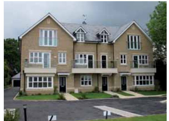
Standard A810 Chamfered Plinth Course, C1 Stooled Cills and GV1 Gable Vents. (WCM)
