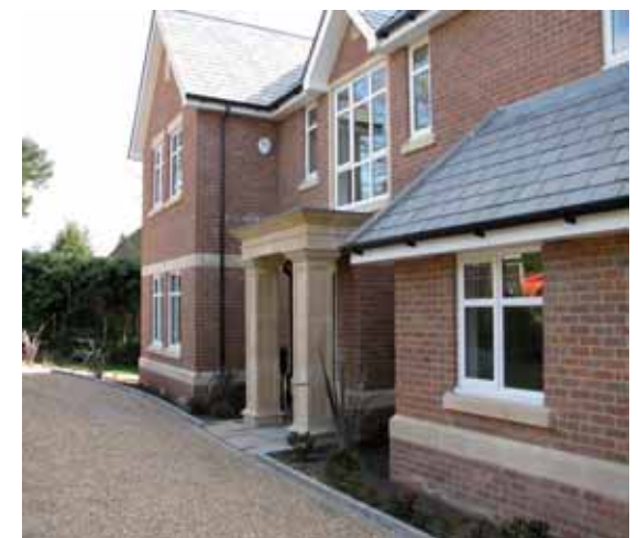
Square Columns with Type C Entablature, A800 Plinth Course, H1 Window Heads, C1 Cills and GV1 Gable Vents. (WCM)
