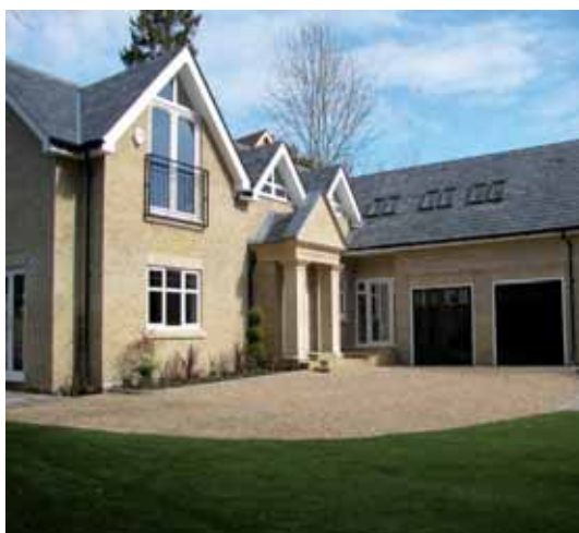
Square Columns with Pedimented Portico produced from Type C Entablature, H1 Window Heads and C1 Stooled Cills. (WCM)
