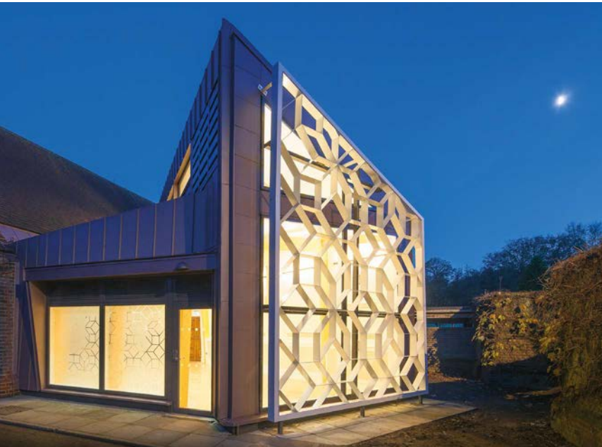
Medway Crematorium, Kent. Renovations designed by Clay Architecture. Sunscreen fabricated by Hellings Fabrications Ltd. Galvanized and powder coated by Joseph Ash Galvanizing.
