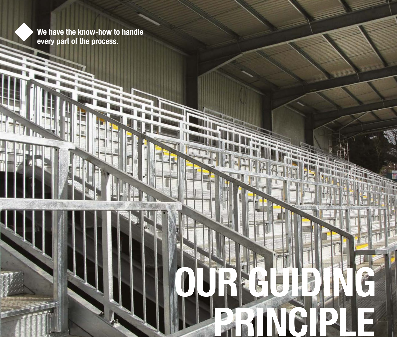
The steel-framed standing terrace at the Gallagher Stadium, galvanized by Joseph Ash for REID Steel.
