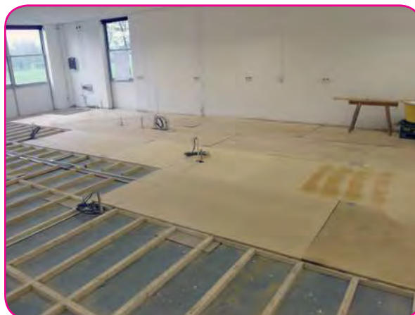
new floor which had to be installed
