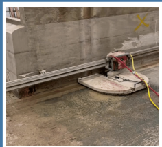
TRACK/WALL SAWING
