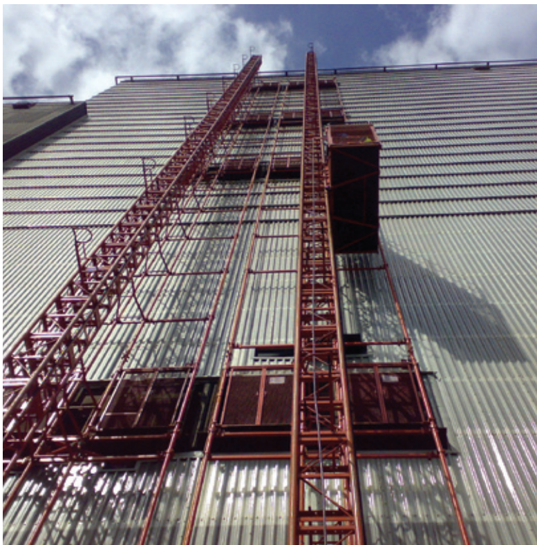
Power station cladding
