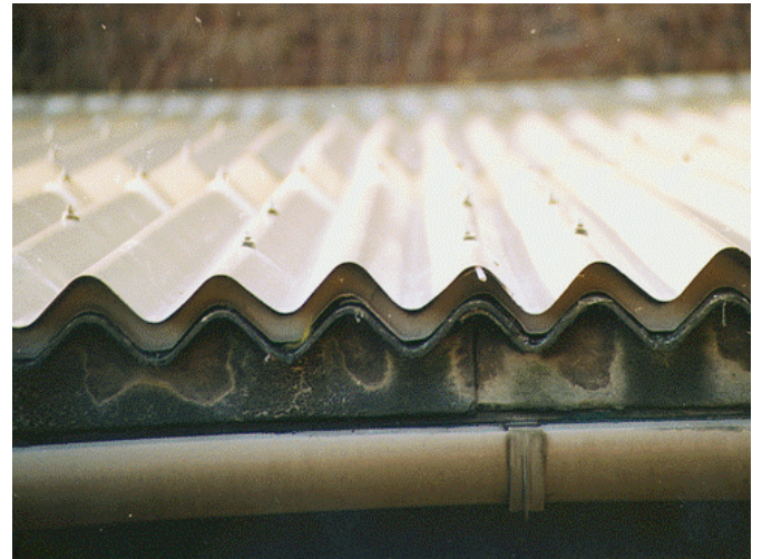
Roof edge detail showing Filon Profix Spacer
